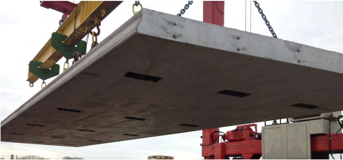
Figure 4.3 – Photo of full size demonstration deck panel showing panel soffit and shear pockets
