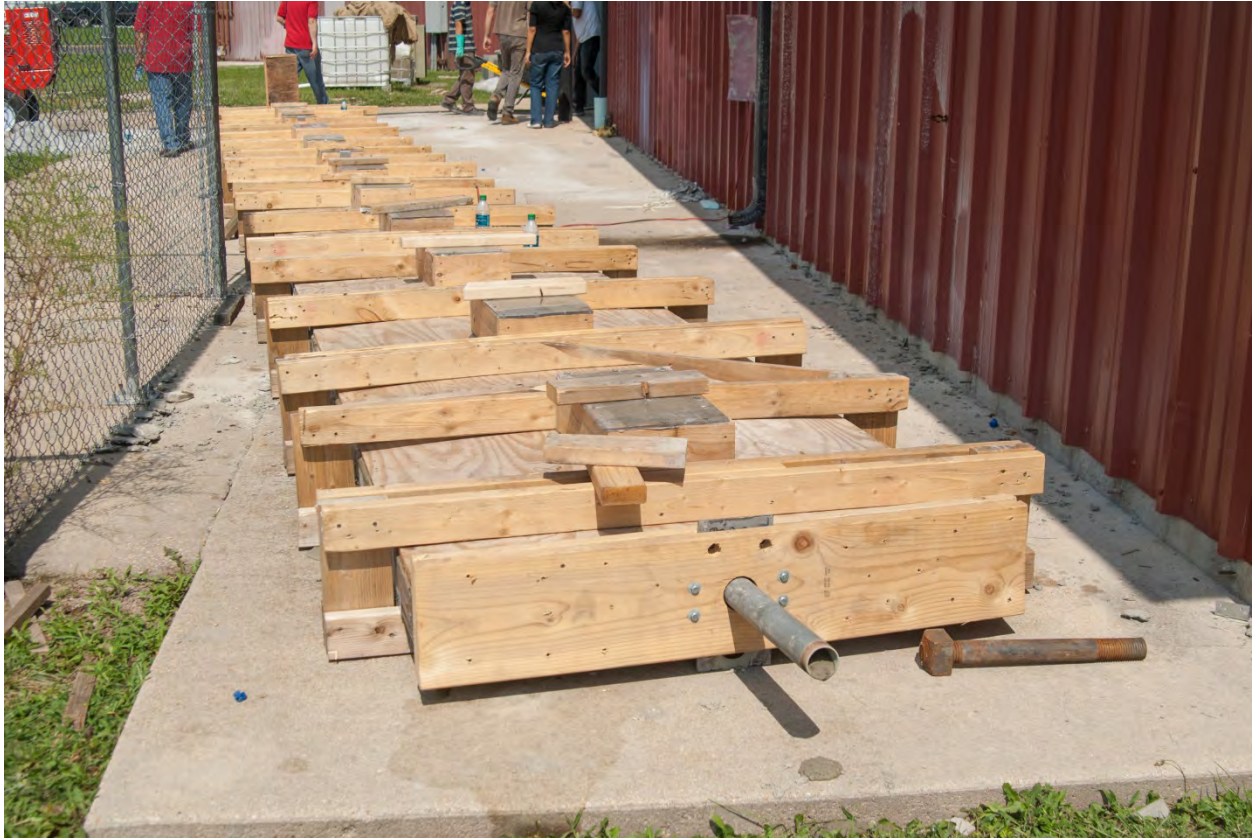
Figure 3.14 – Photo after the completion of casting from both ends
