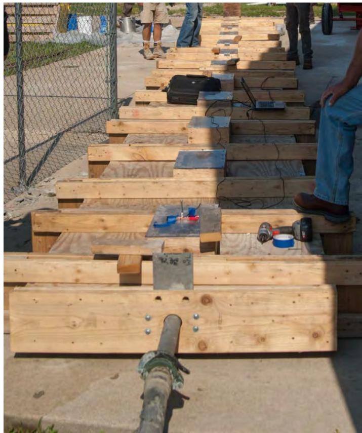
Figure 3.13 – Photo of the second pumping stage
