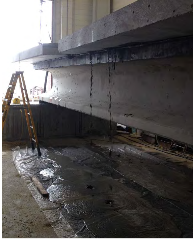
Figure 4.12 – Concrete leakage during pumping due to deck uplift
