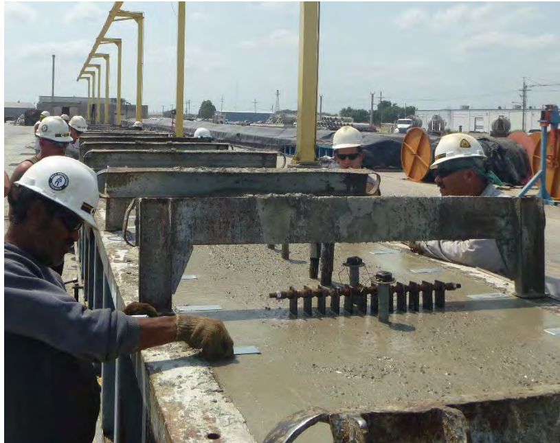
Figure 4.2 – Photos of girder fabrication
