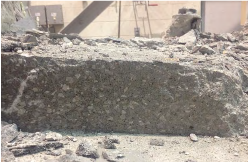
Figure 4.15 – Coarse aggregate distribution in haunch concrete (HVSI = 1.0)
