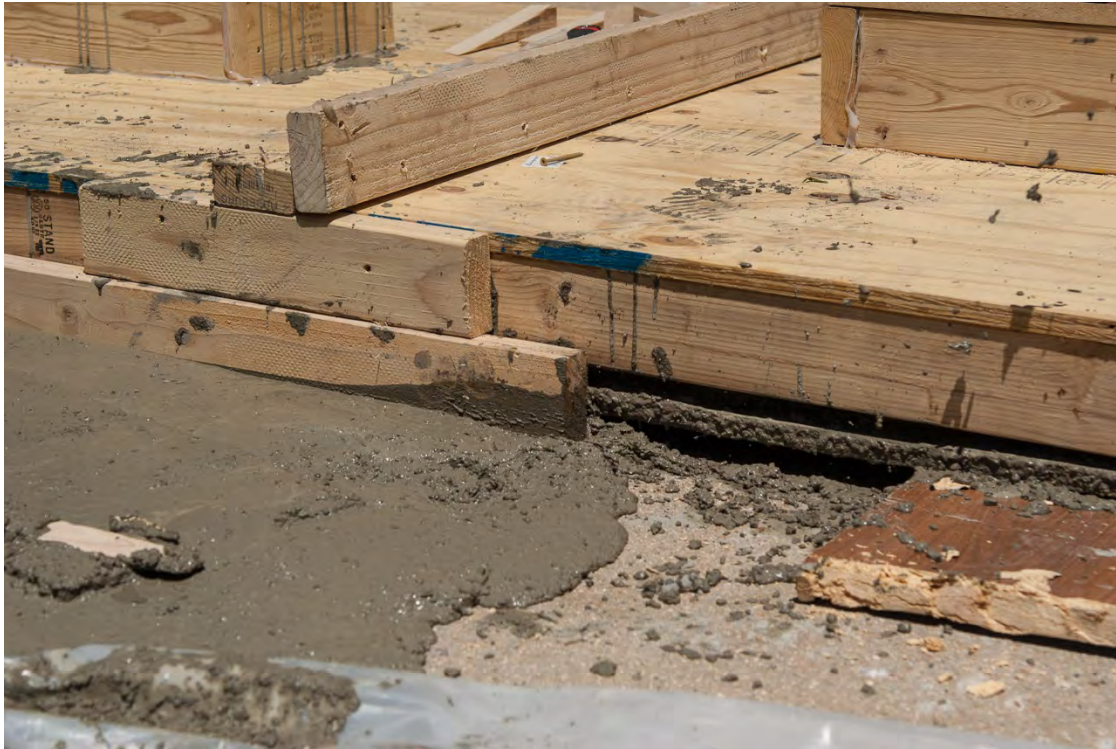
Figure 3.3 – Leakage of concrete after formwork failure due to high concrete pressure at one end
