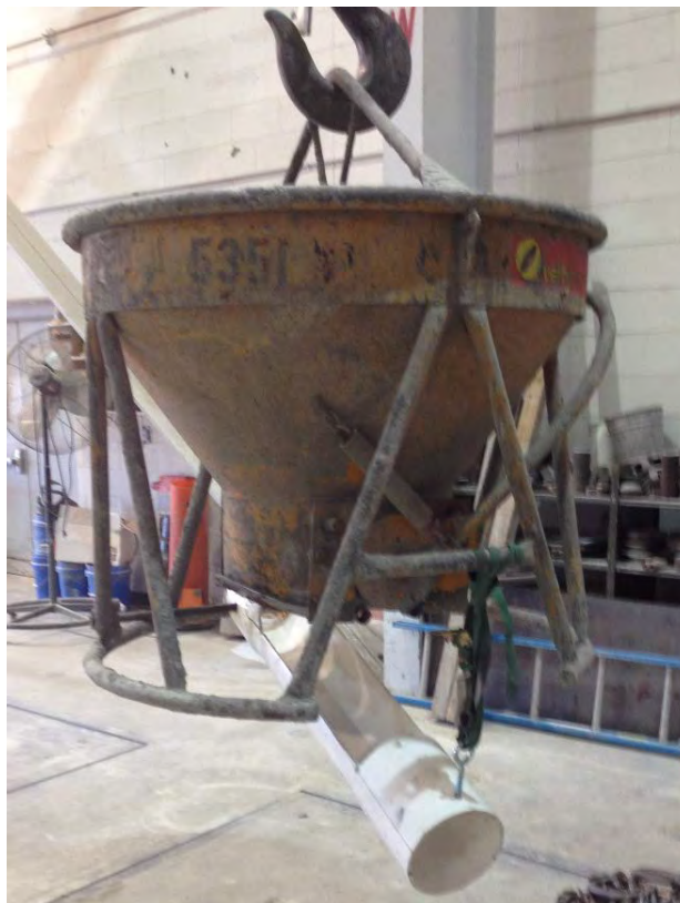
Figure 5.5 – The bucket and chute used in pouring SCC
