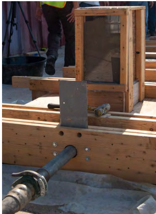
Figure 3.9 – Pumping line connected to the one end of the formwork and concrete pressure indicator tower to monitor pressure build-up exerted on the formwork
