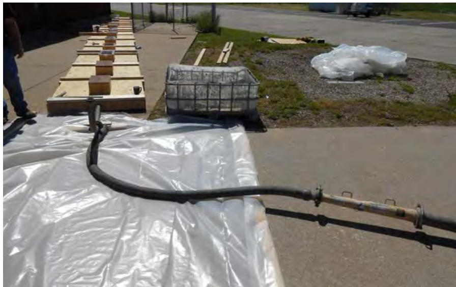
Figure 3.1 – Photo of the formwork and pump connection at one end
