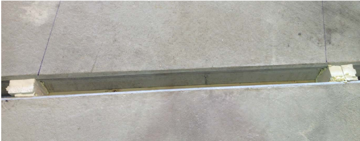
Figure 4.6 – Transverse joint between adjacent deck panels.
