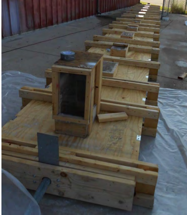
Figure 3.6 – Photo of the formwork, pump connection, and pressure indicator at one end
