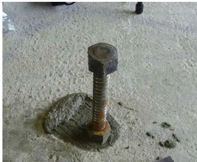
Figure 4.11 – Plugging 1 in. diameter vents
