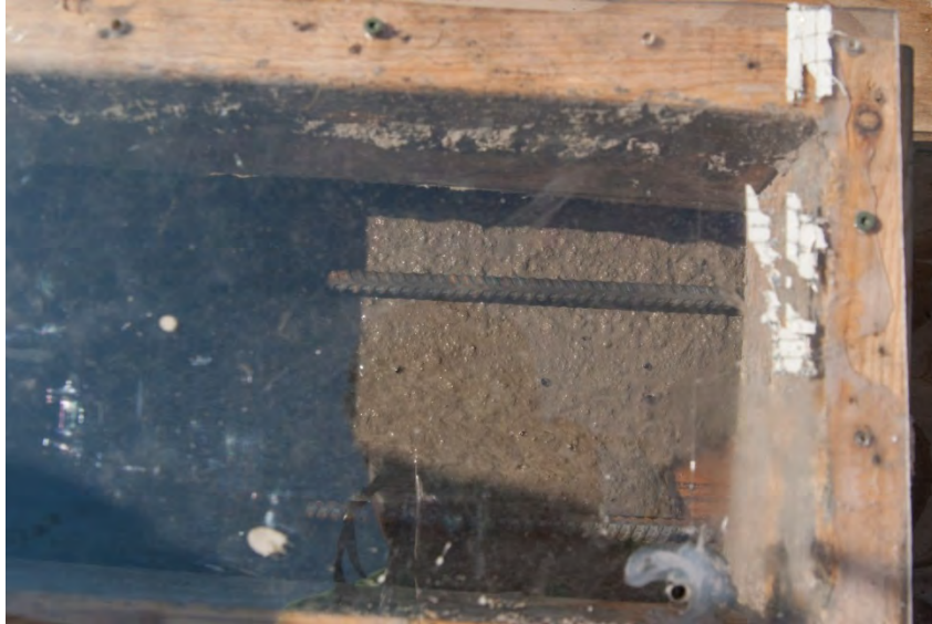
Figure 3.12 – Photo of center of the form after the first pumping stage
