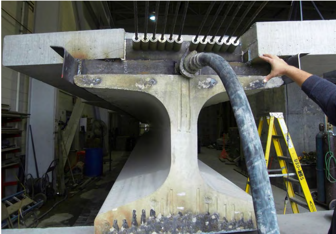
Figure 4.10 – Pumping SCC using 2 in. diameter hose
