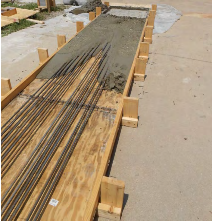
Figure 3.7 – Photo of concrete flow in the field test No. 2 (sudden loss of workability)
